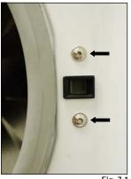
• To remove the Door Switch, remove the two (2) T-15 Torx screws (Fig. 7-1). Then remove the Top Panel as described in Section 2. With the Top Panel removed disconnect the wire harness from the Door Switch and replace (Fig. 7-2).
